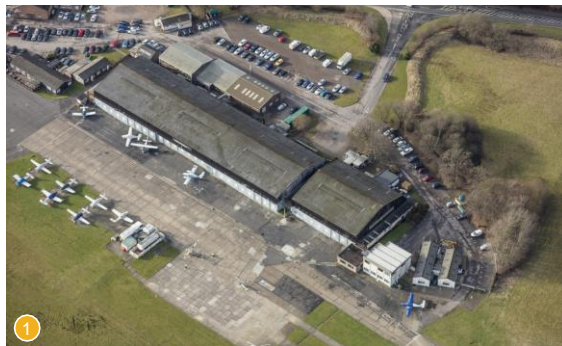
Existing buildings on site with a variety of businesses in operation
