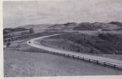
IMPROVED PARK ROADS
